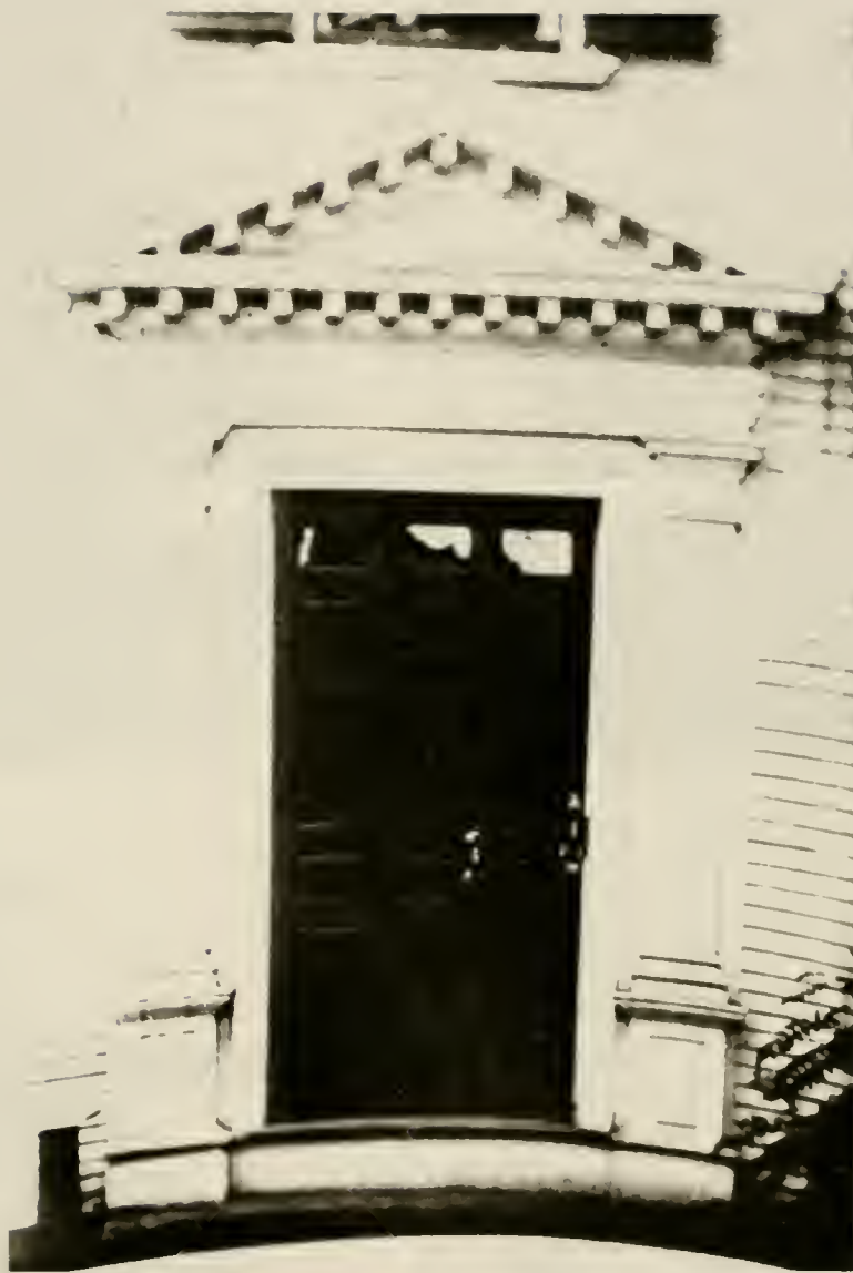
18 Front Entrance Door, Carreth House, Amherst, NH.
